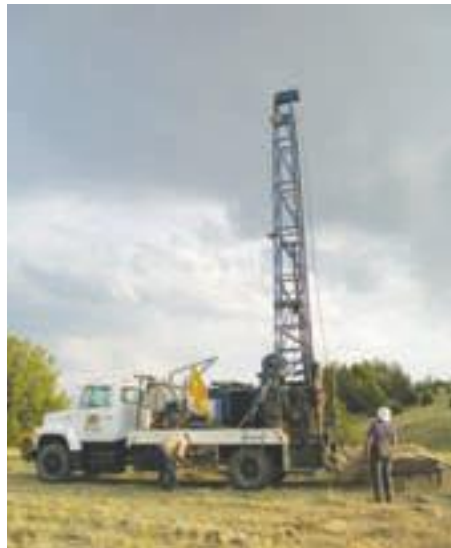
Drilling at New Departure in the US
