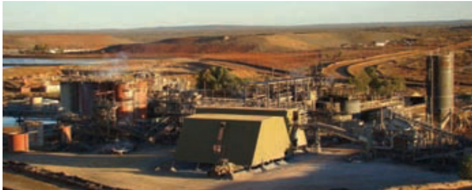
Blackham Resources' Matilda gold mine in Western Australia
